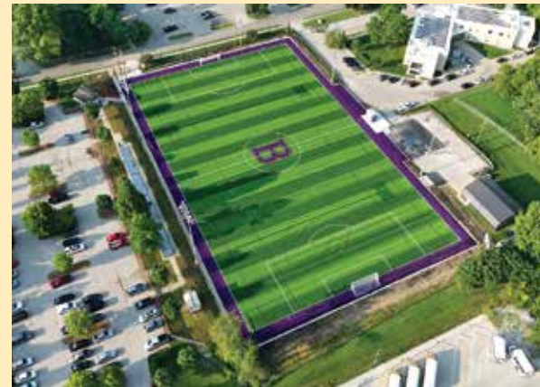
Bloomington High School South’s new soccer field. The school corporation is investing in state-of-the-art facilities through its Designing and Building to Sustain Excellence Initiative. Zero referendum dollars are used in these facilities projects
